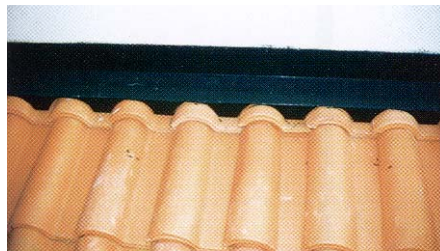
Fig. 90 - Remate com parede transversal emergente
