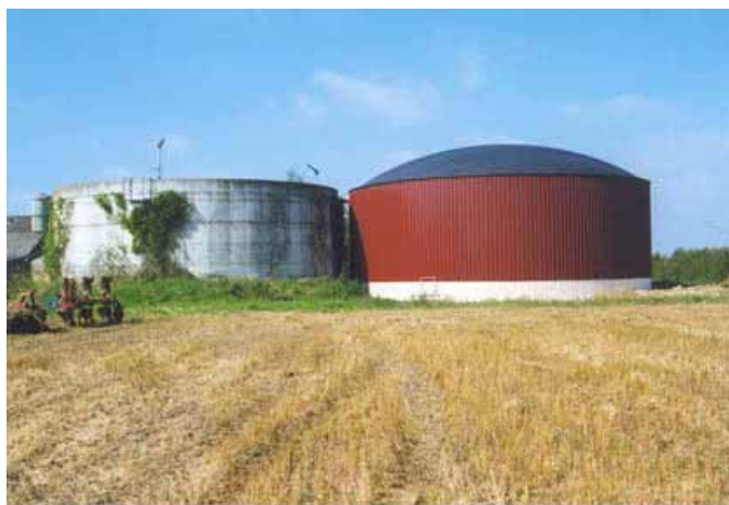
Figura 3.11 - Digestor vertical
